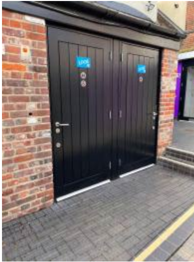
External view of the courtyard accessible toilet (door on the left)
