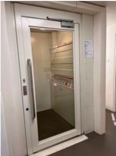
The lift shown from the first floor
