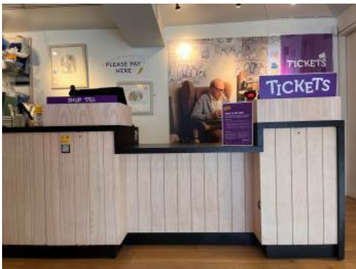
The ticket desk showing the lowered section
