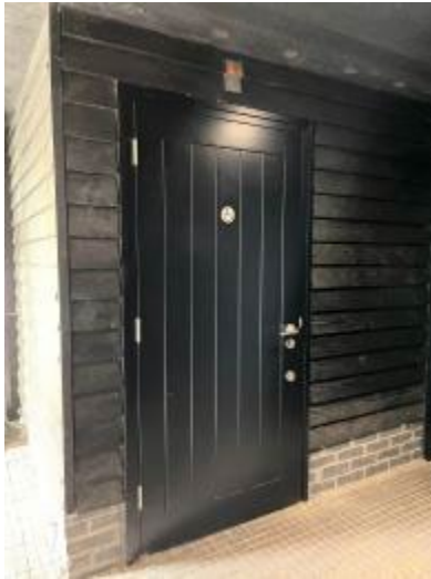
External view of the accessible toilet within the main Museum toilet area
