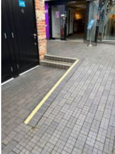
The ramp and steps to access the courtyard accessible toilet
